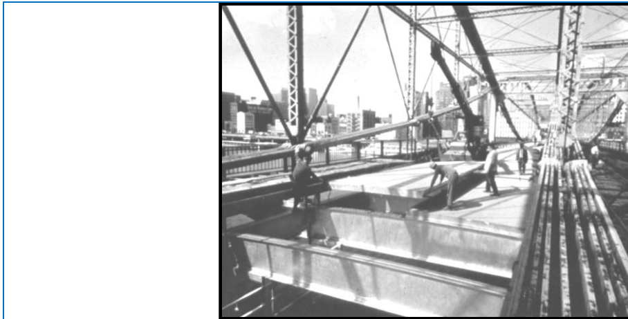
Fig.1 Installation of an aluminum deck on aluminum beams [1]
